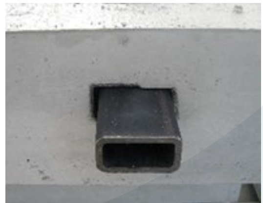
CVS inner part slide out of bearing.
