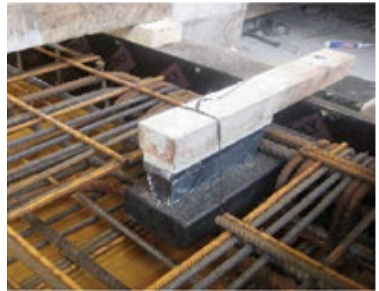
CVS bearing in mold.
